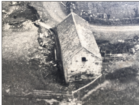
The mill and millwheel.
